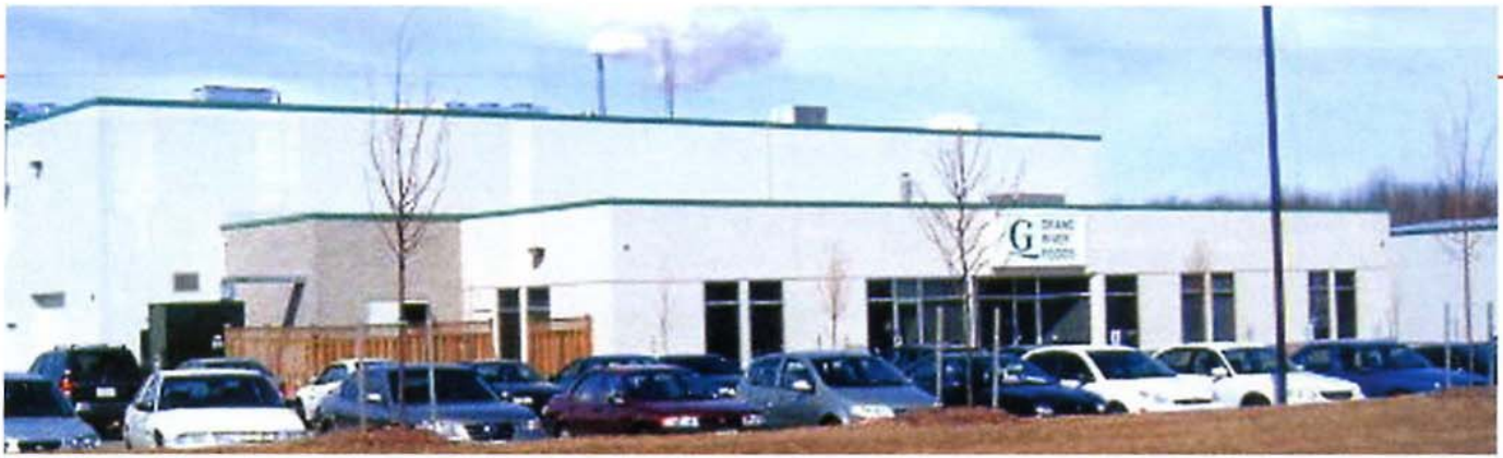
Grand River Foods New Food Processing facility in Cambridge.
