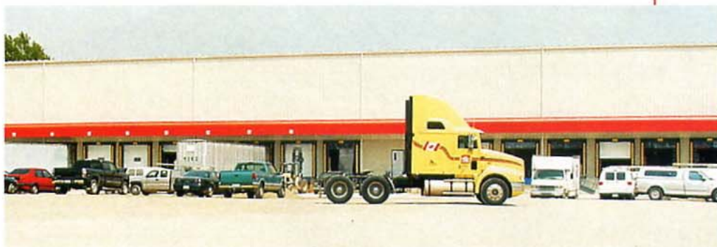
Home Hardware Warehouse Additions, Phases One and Two, in St. Jacobs.
